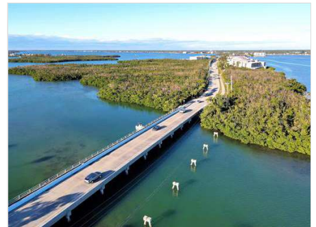
Beach Rd Bridge to Englewood Beach
